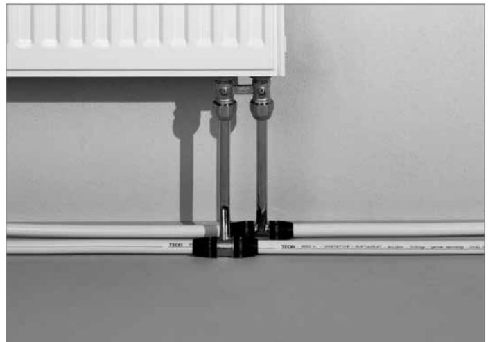
Radiator connection with radiator mounting tee
