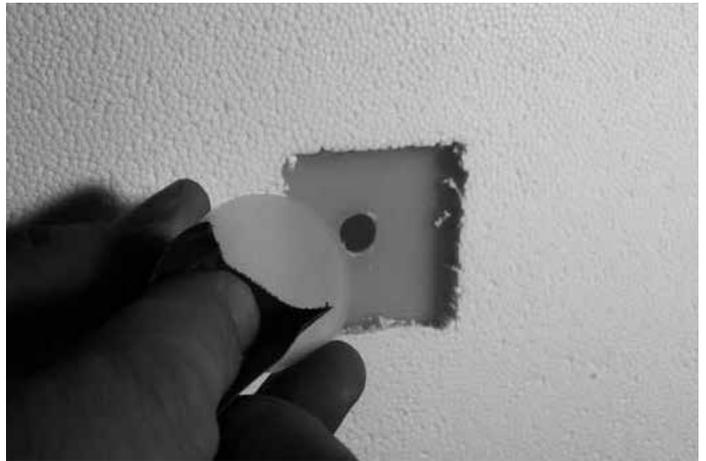
Clean the area to be repaired thoroughly using a solvent or acetone.
